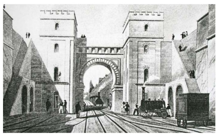
This was the Moorish Arch at Edge Hill pictured shortly after the opening of the Liverpool to Manchester railway in 1830. It marked the point where locomotives gave way to cable-hauled carriages down the steep incline to the Crown Street terminus.
